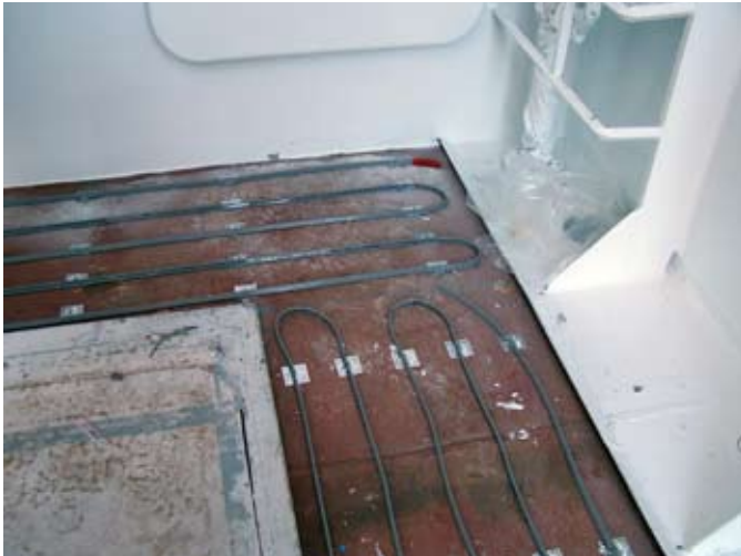
Photo 2: Heating Cable installation on flat surface utilizing brackets with adhesive.
