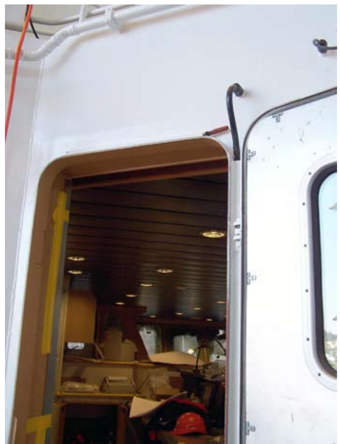
Photo 7: Door frame with Heating Cable installed, power lead and end termination kit shown.
