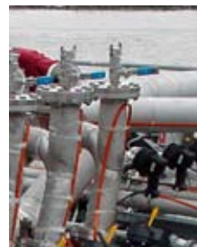
Tanker deck with heat tracing under construction
