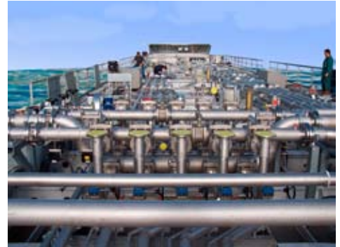
Tanker deck overview
