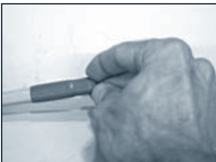
Step 19: Slide the end cap on the end of the cable until fully seated.
