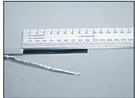
**Step 4:** Cut insulating jacket of cable back 3.5" (90 mm). Wind braid into a pigtail.
