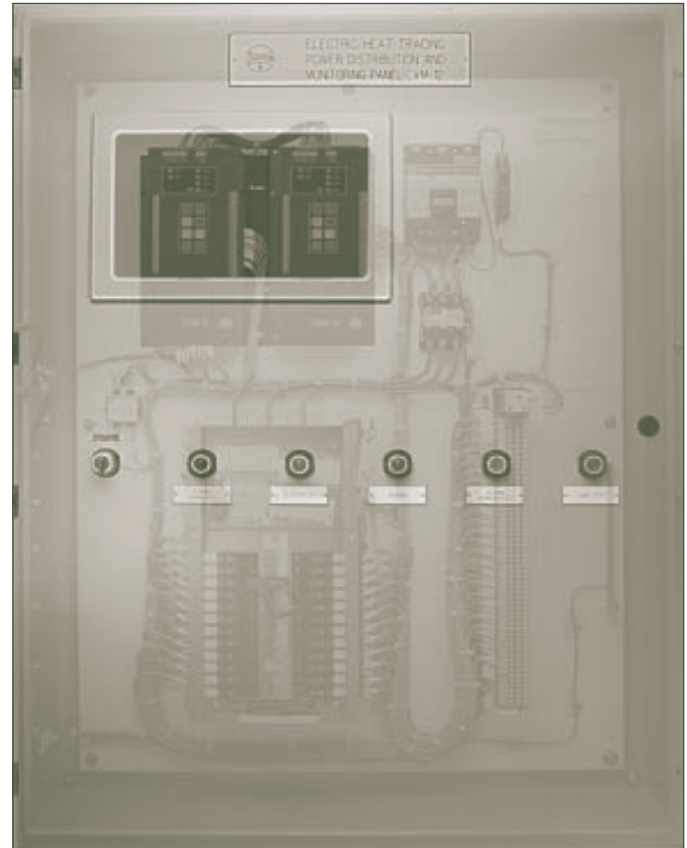
CVM-12 mounted in a NEMA 4 painted steel enclosure
