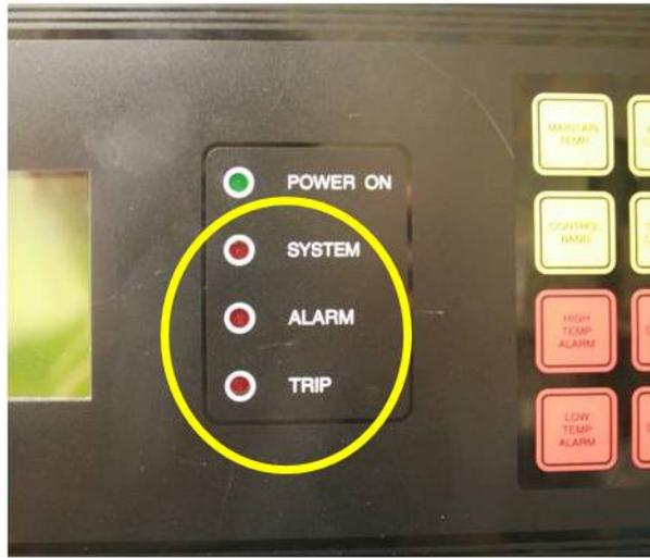
**Figure 10:** Common System, Alarm, and Trip LEDs
