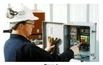
**Figure 4**Mocroprocessor-based monitoring and control units for electric tracing systems — control band programmable in increment of 1 degree.
